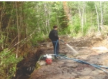
Washing up bedrock before channel sampling at Gosselin
